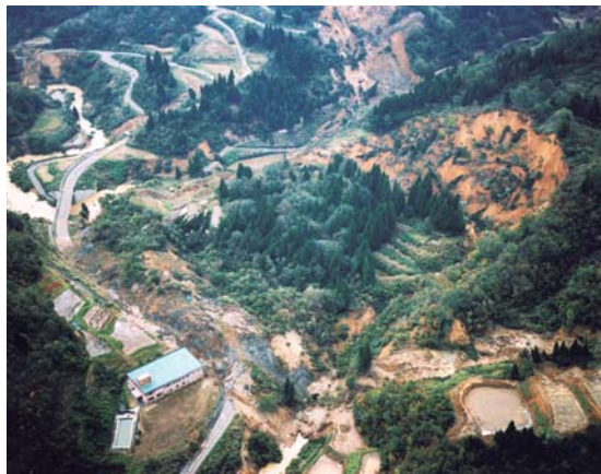
Landslides caused by Chuetsu Earthquake in Niigata Prefecture (2004, Nagaoka City, Niigata Prefecture (Former Higashi Takezawa area of Yamakoshi Village)) Earthquake can cause landslides.
