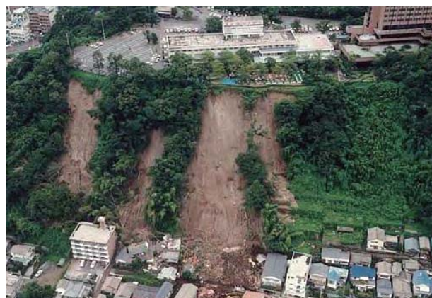
Slope failure of Shirasu terrace (a mass of accumulated volcanic ash) (1986/Kagoshima heavy rainfall disaster, Hirano Town, Kagoshima City, Kagoshima Prefecture)
