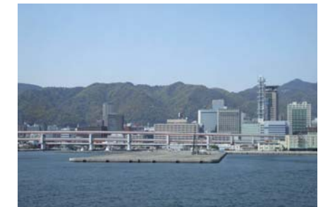
Rokko Mountains at present "Green" has revived after 100 years of the hillside works.
