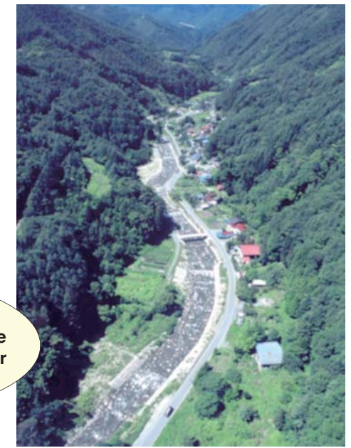
Channel works (Nomugi-Pass channel works, Matsumoto city, Nagano Prefecture) Parks constructed along the river.
